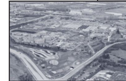
South Treatment Plant, Renton
