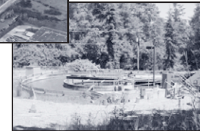
Vashon Island Treatment Plant
