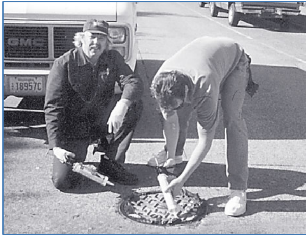
Sometimes odor prevention solutions can be as simple as resealing a manhole cover. Other problems can be more complex.
