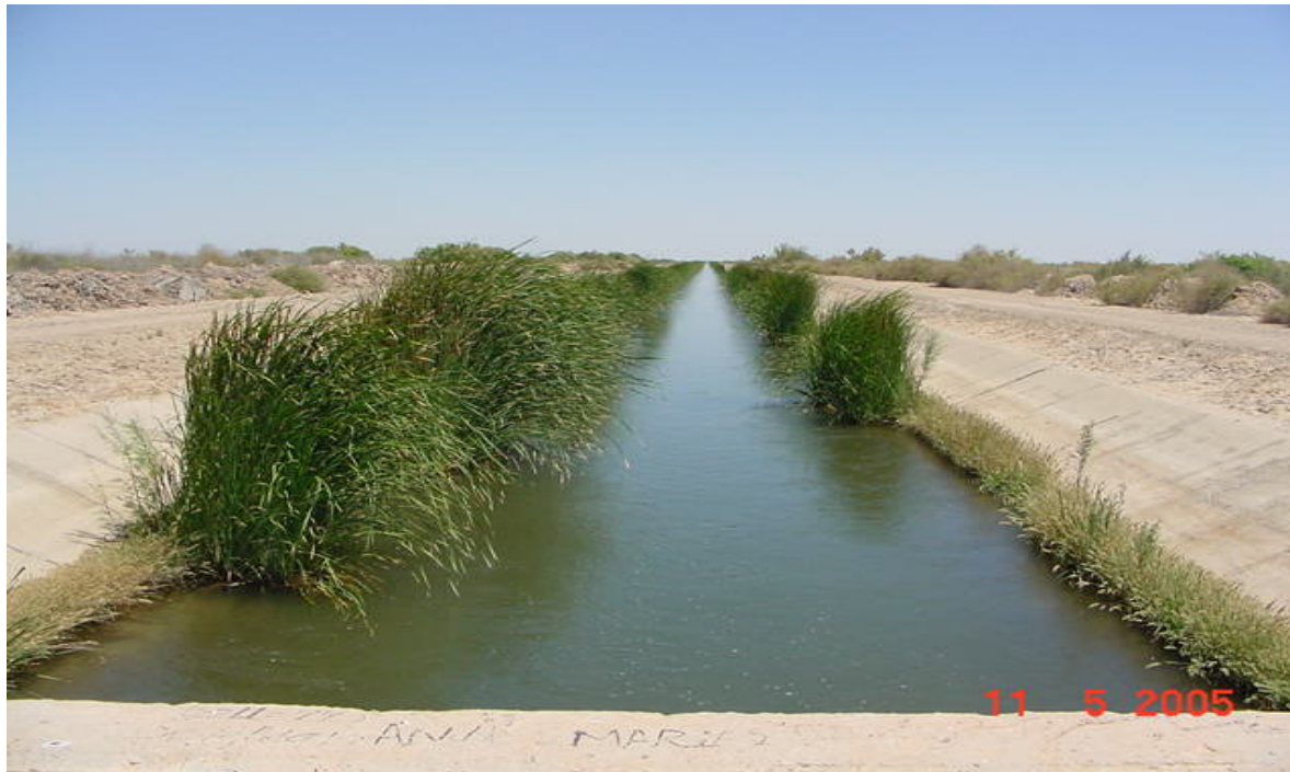
Wellton Mohawk Bypass Drain
