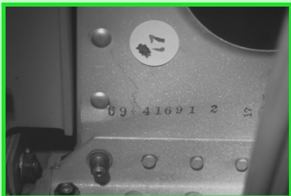
Crack Removed Image
