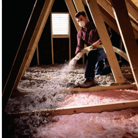
Use a blowing machine to blow in loose fill insulation.
