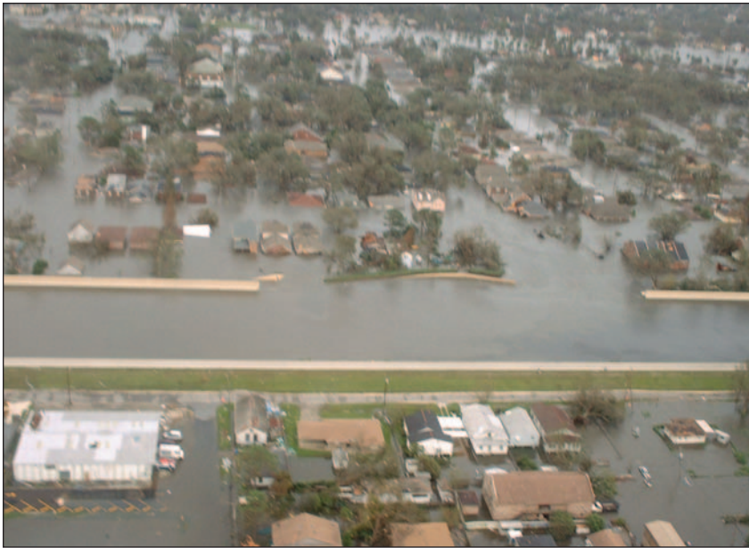
Breached floodwall, New Orleans Marty Bahamonde photo
