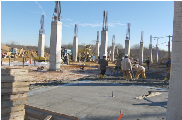
Caption: Footings and concrete "slab on grade" (SOG).
