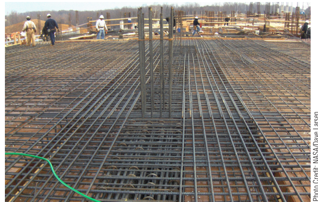
Caption: Rebar reinforcements.
