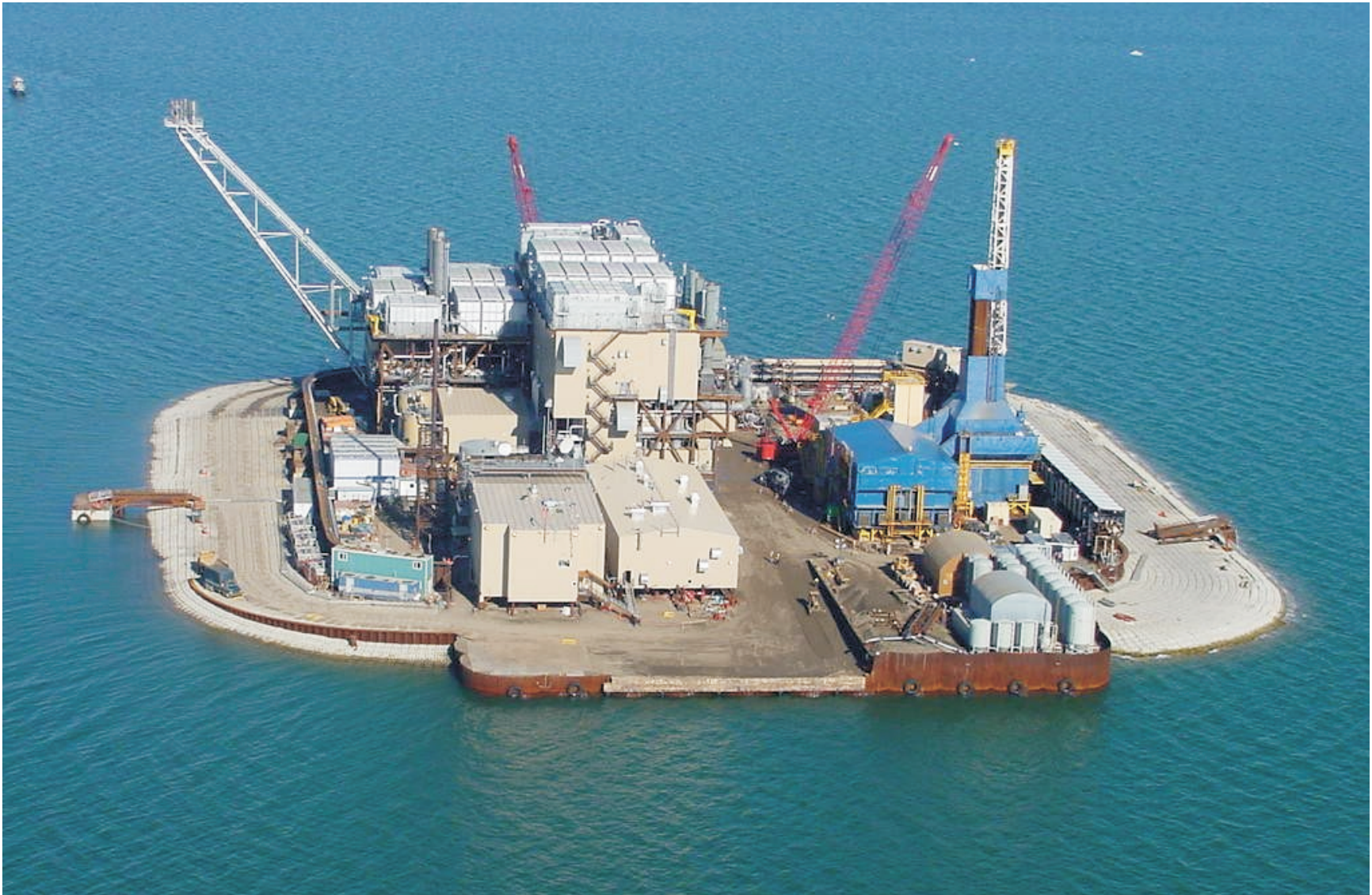
Fig. 3 Northstar Island looking north, September 2001. Production started in November 2001.
