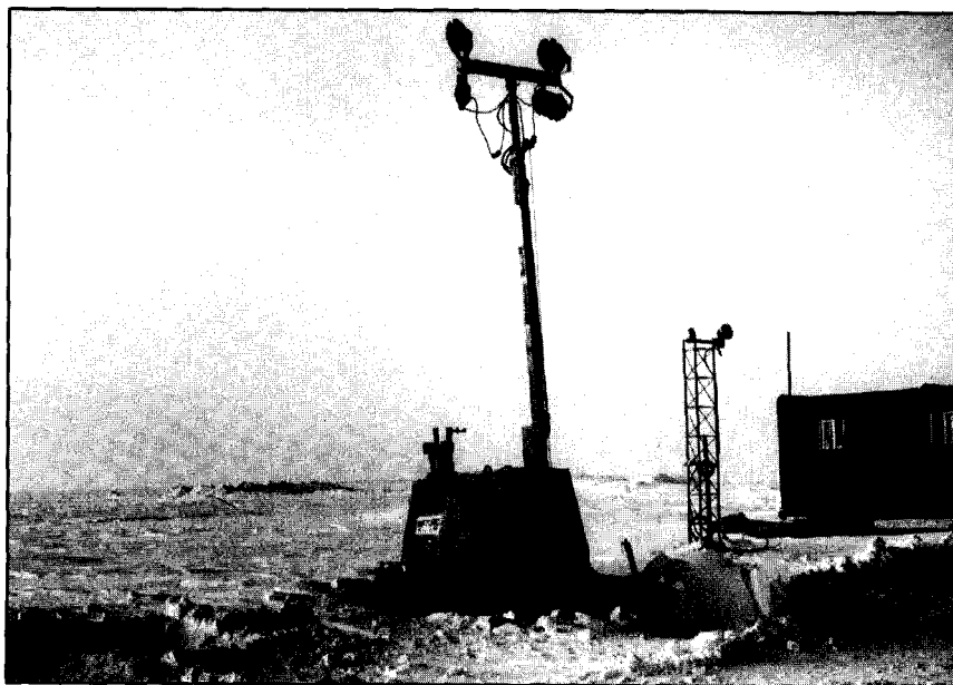
Figure 4-2. Exterior alarm (strobe and horn mounted on tower) and floodlights facing outward toward trip wire were part of CONOCO's detection system at "Badami II" drillsite (D. Shideler).
