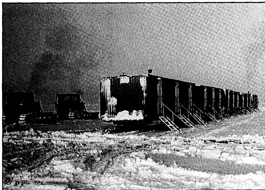
Figure 8-8. Seismic operations, being mobile, cannot always be equipped with skirting around buildings (W. Sands).
