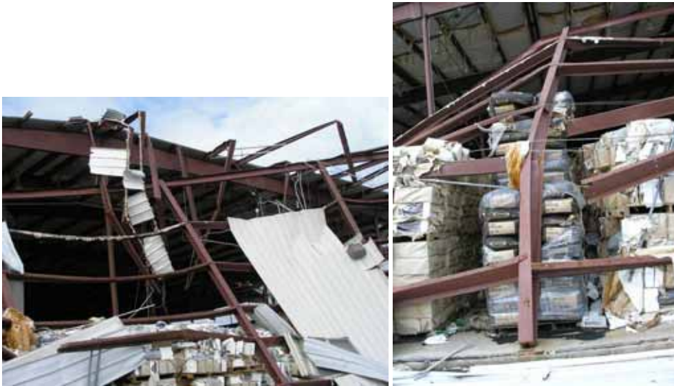
Figure 3-15 Collapse of the entire end bay of a steel-frame warehouse from wind pressure near Long Beach, MS (Photo credit: NIST).
