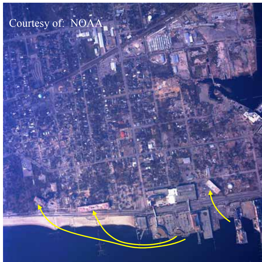
Figure 3-19 Movement of three casino barges that broke completely free from their moorings and were deposited inland (Photo credit: NOAA).
