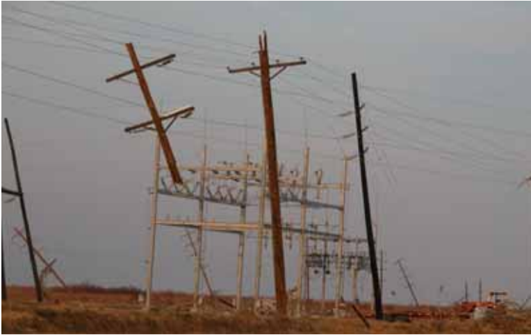
Figure 4-71 Distribution lines on US Route 82 in Louisiana damaged by Hurricane Rita (photo credit: NIST)
