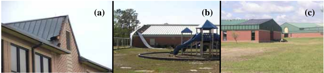
Figure 3-34 Limited damage to standing seam metal roofs at (a) Lamar State University in Orange, TX (Photo credit: Dominic Sims), (b) at Gulfview Elementary School near Waveland, MS (Photo credit: NIST), and at (c) Hancock High School in Kiln, MS . Damage occurred at the edge of the roofs along the windward sides of the buildings (Photo credit: Robb Smith, Amtech Roofing Consultants).
