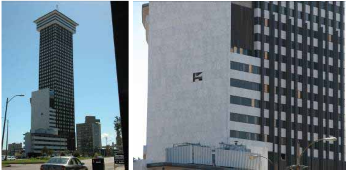
Figure 3-51 Unusual instance of damage to stone cladding due to wind pressure (Photo credit: Keith Porter, Scawthorn Porter Associates).
