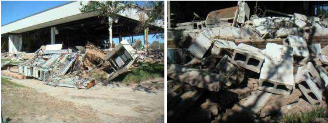
Figure 3-4 Storm-surge-induced collapse of CMU walls at the Venetian Isles Fire Station in New Orleans (Photo credit: Keith Porter, Scawthorn Porter Associates).
