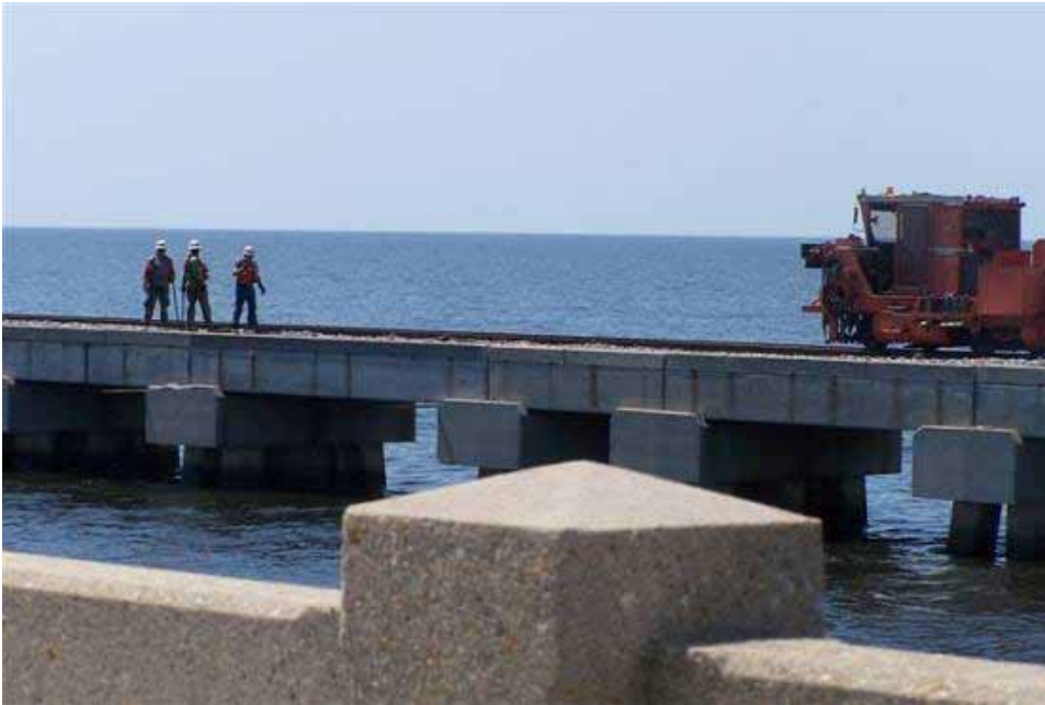
Figure 4-33 The Norfolk Southern Railroad bridge over Lake Pontchartrain had its tracks stripped from the superstructure but otherwise remained intact (photo credit: J. O'Connor, MCEER).
