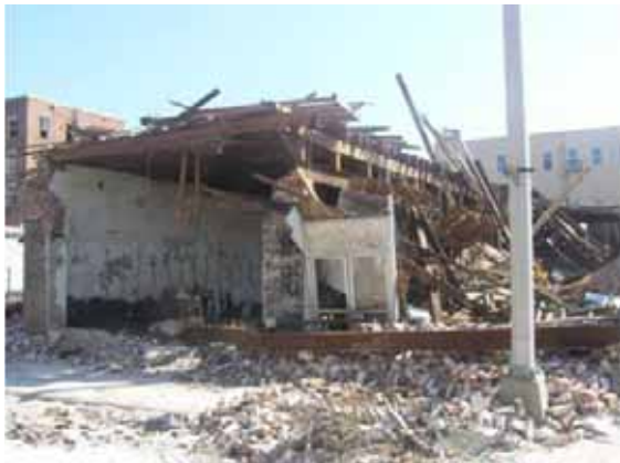
Figure 3-13 Collapsed unreinforced masonry building in downtown Gulfport, MS (Photo credit: NIST).
