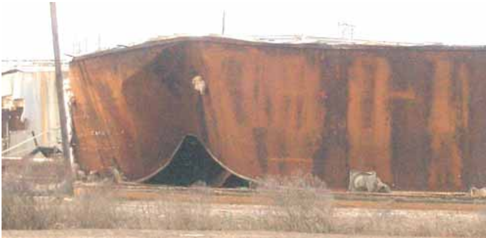
Figure 4-79 Buckled oil storage tank in Port Sulphur, LA (photo credit: Keith Porter, Scawthorn Porter Associates)
