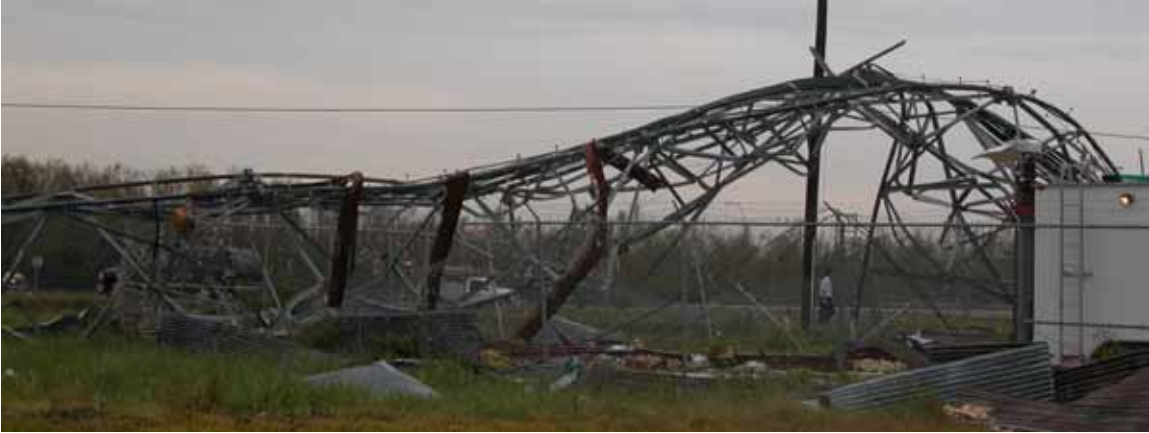
Figure 4-76 Cell tower downed by Hurricane Rita, in Orange, Texas (photo credit: NIST)
