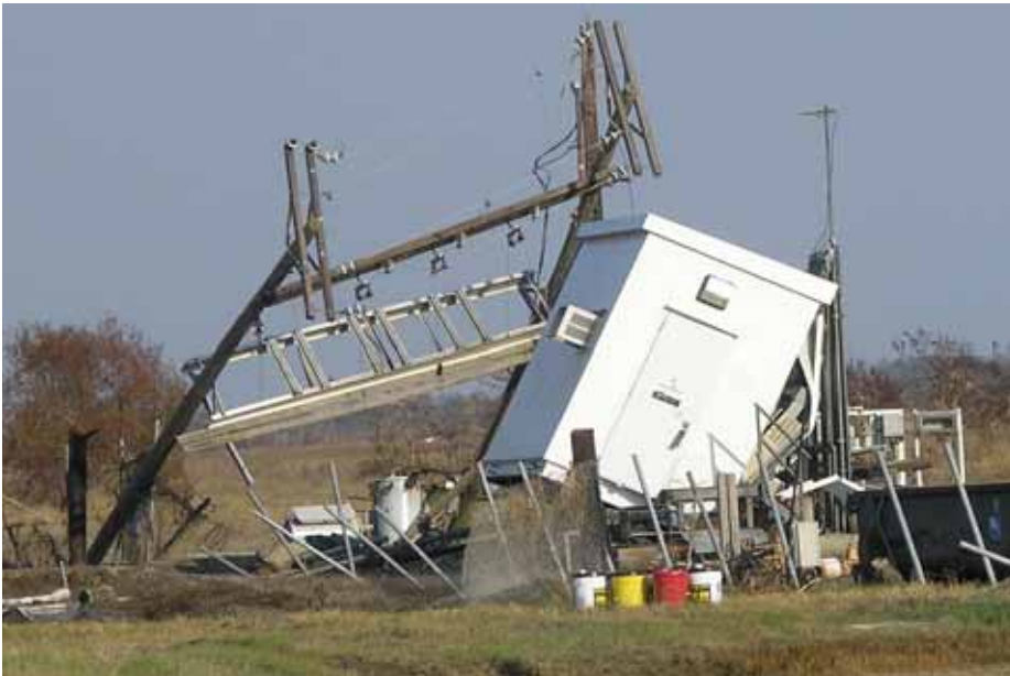
Figure 4-72 Substation damaged by surge and waves on US Route 82 in Louisiana following Hurricane Rita (photo credit: NIST)
