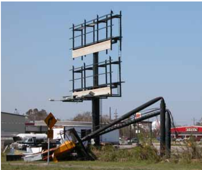
Figure 4-69 Typical billboard failures along US Interstate 10 near Beaumont, Texas (photo credit: NIST)
