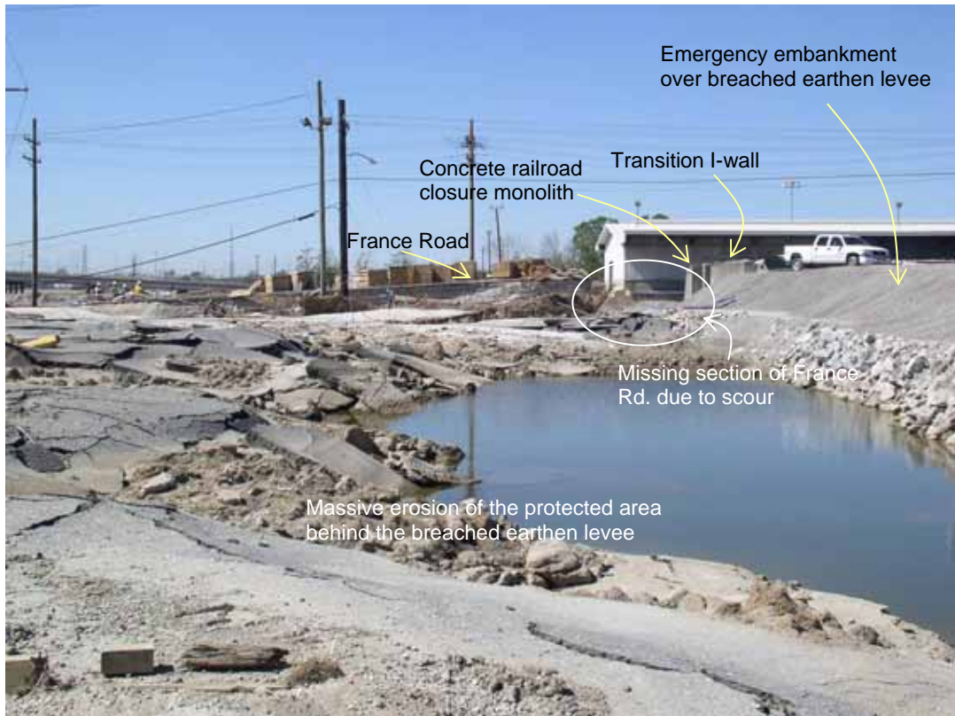
Figure 4-21 Erosion behind breached earthen levee. The breach occurred at the transition between the earthen levee and the transition I-wall (photo credit: NIST)
