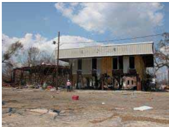
Figure 3-17 Damage to a metal building in Gulfport, Mississippi (Photo credit: Keith Porter, Scawthorn Porter Associates).
