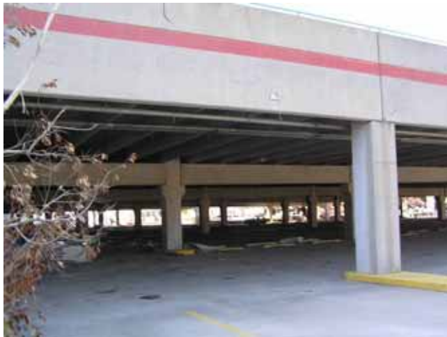
Figure 3-2 Successful performance of a single-story parking structure in Biloxi, MS (Photo credit: NIST).
