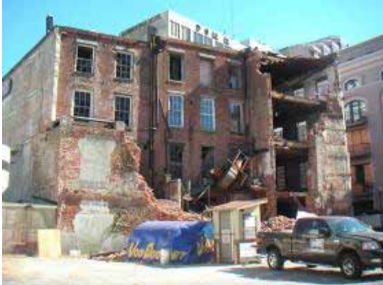
Figure 3-11 Partial failure of a load-bearing masonry wall in New Orleans, LA (Photo credit: NIST).
