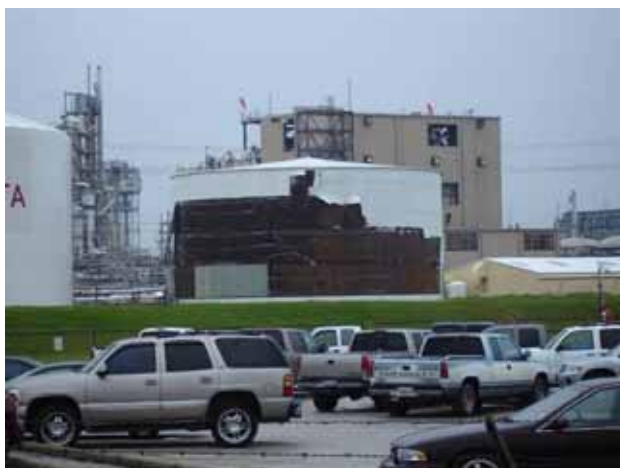
Figure 4-78 This tank at the Dupont Sabine River Plant in Orange, Texas, lost its wall insulation in Hurricane Rita (photo credit: NIST)
