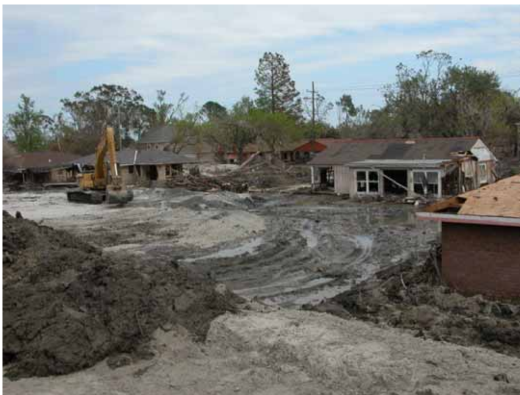
Figure 5-11 Destruction of residential structures near the London Ave Outfall Canal breach in New Orleans. (Photo credit: Keith Porter, Scawthorn Porter Associates)
