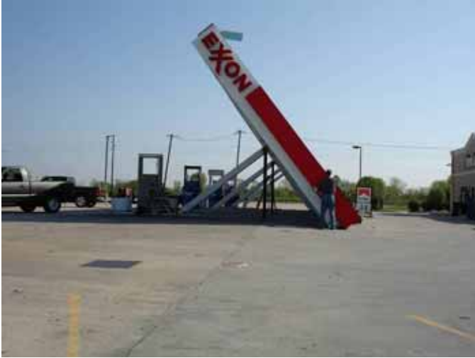
Figure 4-81 Gas station near Port Arthur, Texas with column failure (photo credit: NIST)
