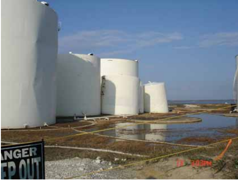
Figure 4-80 Shifting of oil storage tanks, Monroe Petroleum plant, Biloxi, MS. (photo credit: D. Fratta, U. of Milwaukee)
