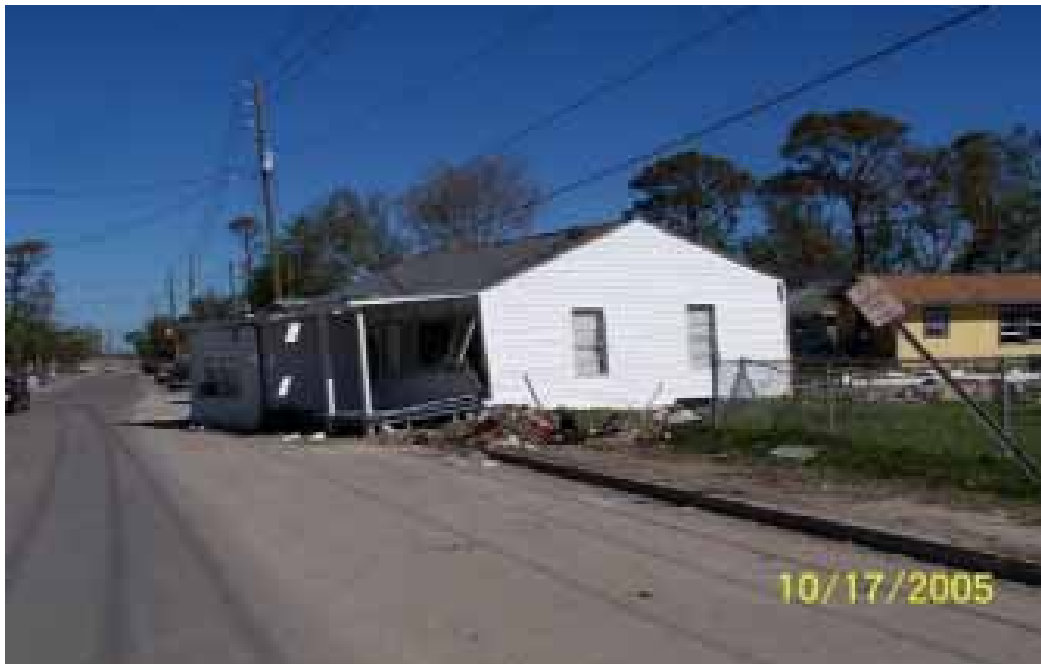
Figure 5-10 A single-family residential structure in downtown Biloxi was pushed or floated off its low foundation. (Photo credit: Thomas B. Rodino, Shiner Moseley and Associates, Inc.)
