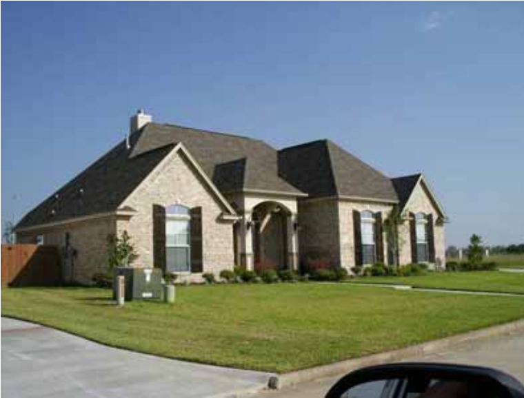
Figure 5-23 Home with undamaged laminated asphalt shingles estimated to be less than 5 years old, Beaumont, TX. (Photo credit: NIST)
