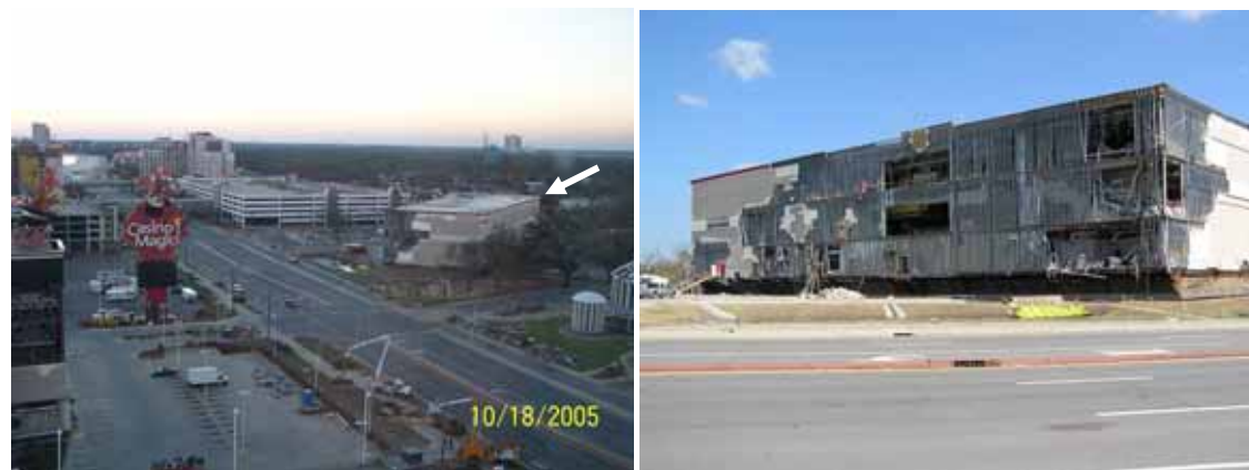
Figure 3-20 Casino barge (arrow) in Biloxi, MS, broke free of its mooring and floated about one-quarter mile inland (Photo credit: NIST).
