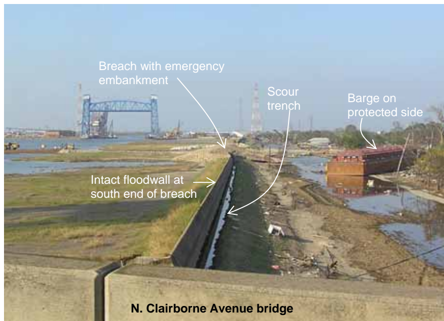
Figure 4-24 View looking north at the IHNC Lower Ninth Ward South breach (photo credit: NIST)
