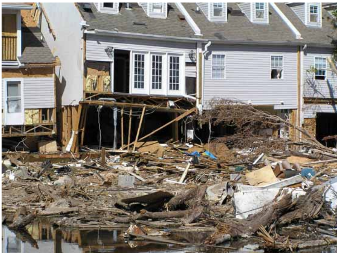
Figure 5-4 Severe damage and destruction to townhomes in Gulfport, Mississippi. (Photo credit: NIST)
