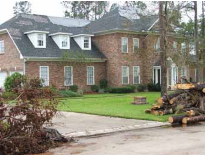
Figure 5-19 Damage to laminated asphalt shingles in Orange, TX. Shingles were temporarily repaired with tarps and roofing felt. No shingle debris was found throughout this and many other neighborhoods. (Photo credit: Dominic Sims, International Code Council)
