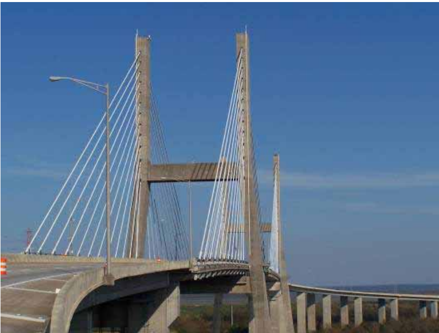
Figure 4-52 The Cochrane-Africatown USA bridge was hit by an oil rig that had been swept to Mobile Bay by Hurricane Katrina's surge. The impact displaced the bridge spans by four inches, necessitating the restriction of traffic on the bridge (photo credit: LA DOTD, provided by J. O'Connor, MCEER).
