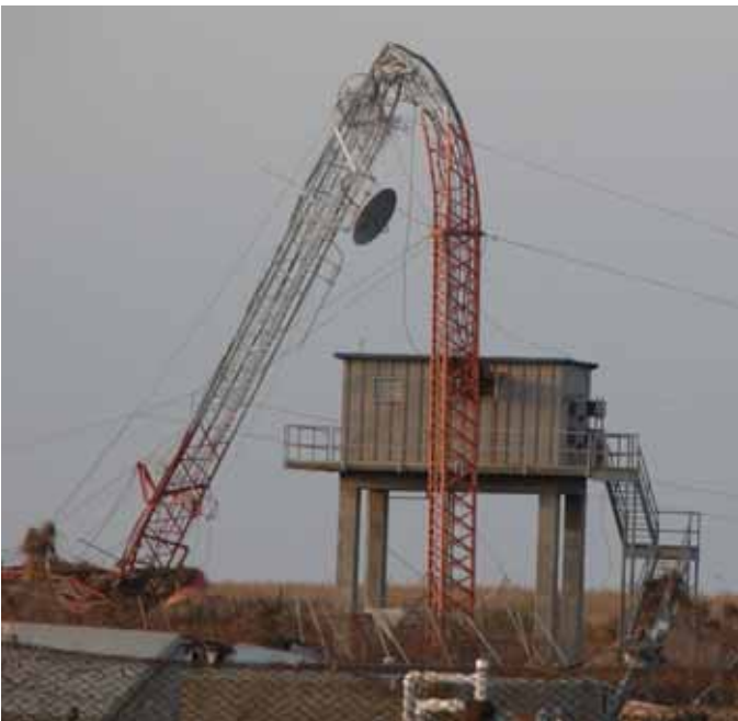
Figure 4-77 Downed communications tower on US Route 82 near Holly Beach Louisiana following Hurricane Rita (photo credit: Christopher Letchford, Texas Tech University)
