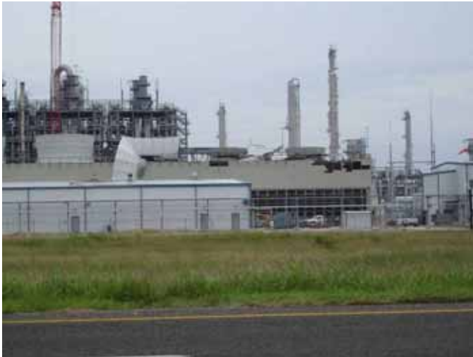
Figure 4-83 Cooling tower failures at the BASF Fina Plant in Port Arthur/Groves, Texas (photo credit: Christopher Letchford, Texas Tech University)
