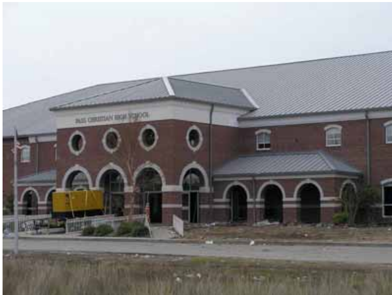
Figure 3-33 Standing seam metal roof in the coastal region of Pass Christian, MS, that sustained Hurricane Katrina without damage (Photo credit: NIST).
