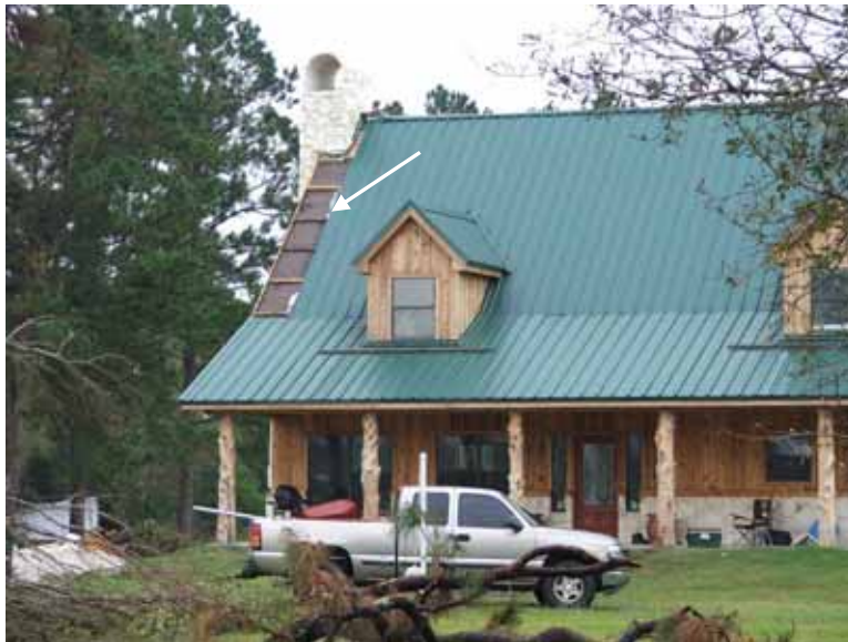
Figure 5-25 Damage to metal roofing (arrow), Orange, TX. Overall, little damage was seen to metal roofing; where seen, it was limited to a relatively small area of the covering and often along an edge of the roof. (Photo credit: Dominic Sims, International Code Council)
