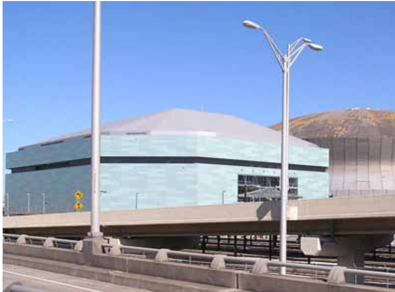
Figure 3-25 The New Orleans Arena, which has an SBS modified bitumen membrane, withstood the Hurricane Katrina winds without damage. (Photo credit: Robb Smith, Amtech Roofing Consultants).
