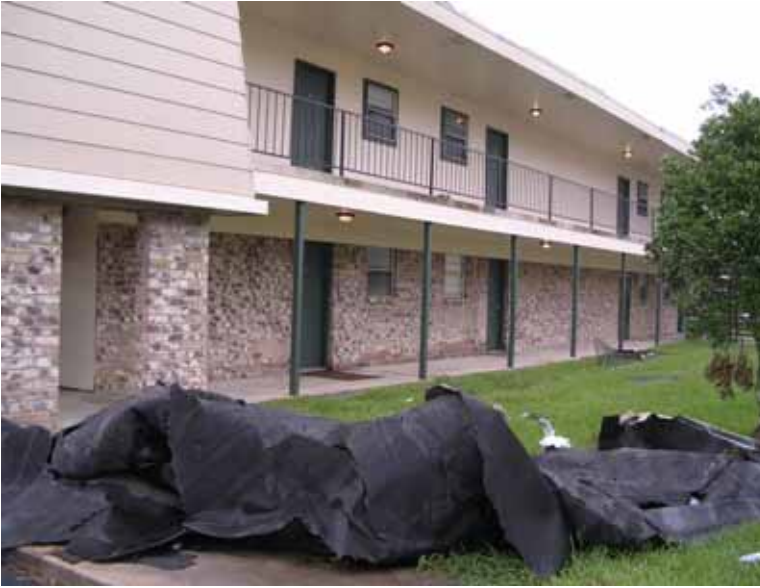
Figure 5-27 Blown-off polymer-modified bituminous membrane at an apartment complex in Orange, TX. (Photo credit: Hua He, Texas Tech University)
