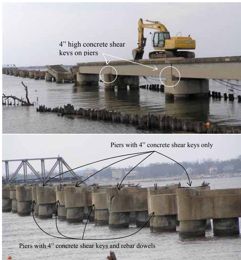
Figure 4-40 CSX railroad bridge with remaining spans (top) and the supporting piers (bottom) (photos credit: NIST).
