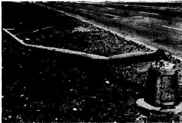
Photograph 48—Collapsed steel lighting standard on U.S. Route 87. View looking north. (Location 28)
