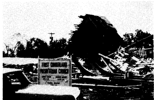
Photograph 7—Church of timber construction. View looking northwest. (Location 6)
