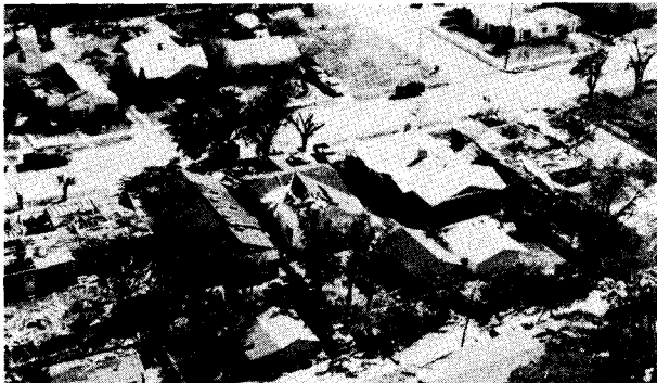
Photograph 5—Random damage to gable roofs of wood framed houses. View looking south. (Location 4)
