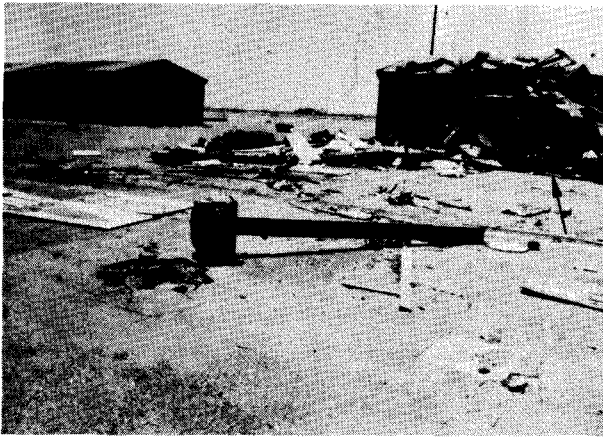
Photograph 61—An overturned steel column is all that remains of several private airplane hangars on the east side of Lubbock Municipal Airport. (Location 33)
