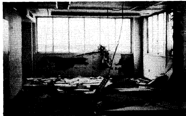
Photograph 24—Southwest corner on the sixth floor of Great Plains Life Building. The 3-inch gypsum tile non-loadbearing walls were shattered by wind pressure. (Location 13)
