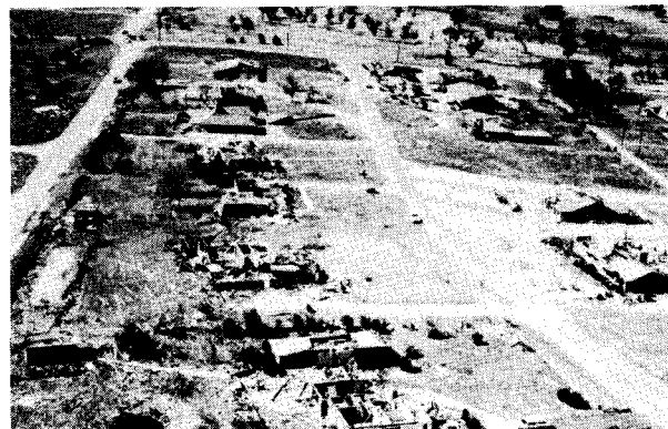
Photograph 54—View looking north on destruction of expensive housing which was in the direct path of the tornado. Note that one house (upper left) in this line escaped damage. (Location 31)
