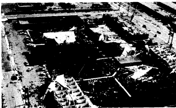
Photograph 1—Apartment complex with considerable loss of structural roof deck. View looking south. (Location 1)
