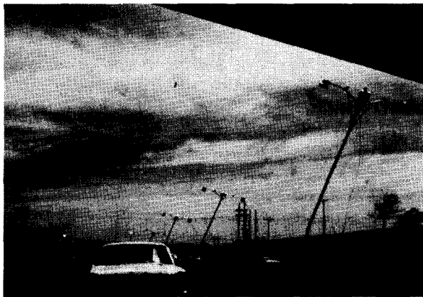
Photograph 49—Median strip lighting standards leaning to the north on U.S. Route 87. (Location 29)
