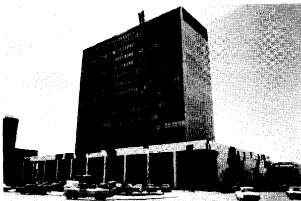
Photograph 9—View of First National-Pioneer Building looking southeast. Glazing, spandrel glass veneer and marble veneer severely damaged. (Location 7)
