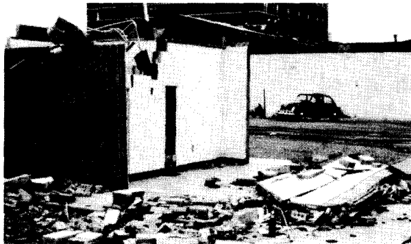
Photograph 16—Small office building for dealer in used automobiles. Roof structure completely removed and non-reinforced masonry walls badly damaged. (Location 9)
