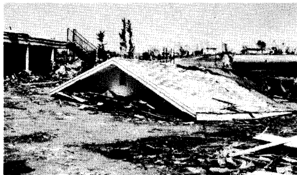
Photograph 46—Complete wood frame roof sucked from the forecourt building of the Ramada Inn Motel and transported 40 feet. (Location 27)
