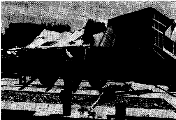
Photograph 58—Mobile home park at Purdue Street with one unit dislodged from its chassis and partly overturned. (Location 32)
