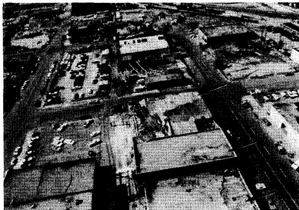
Photograph 36—Roof damage to light industrial buildings. View looking north. (Location 20)
