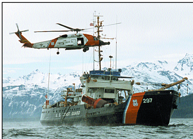
The cutter Ironwood (WLB 297) and an HH-60J offload equipment for maintenance on Eldred Rock Lighthouse, Lynn Canal, Alaska.
