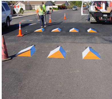
3D markings are holographic images that help curb speeding by giving the illusion of an object in the street.
