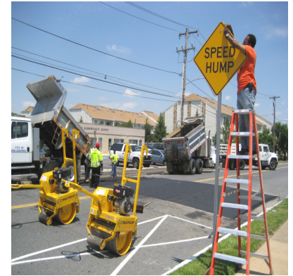
First ever speed humps and 3D markings have been installed on the 900 block of Blue Grass Road, along with new signage to encourage motorists to slow down.
