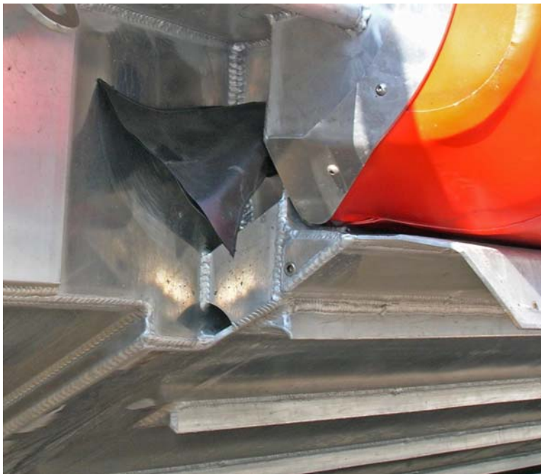
Figure 3-29 Aft Weather Deck Scupper/Water Sock
