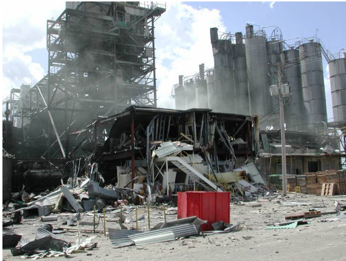
Figure 5. Damage to the Safety and Engineering offices
