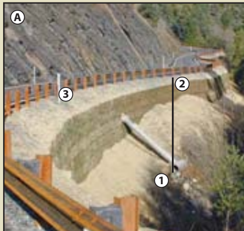
Figure 11.2 – If no records exist for the original photo locations, then a close approximation can be determined (after Hall 2002a). If the photographs were taken along a roadside, it is often possible to relocate the approximate point the photograph was taken by locating permanent structures (such as guardrails and culverts).
