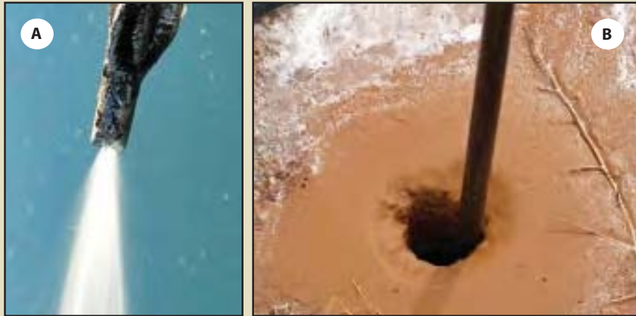
Figure 10.110 – The Waterjet Stinger (A) injects high-pressure water into the soil, turning it to a slurry (B) into which a live stake can be inserted (Photos courtesy of Chris Hoag).
