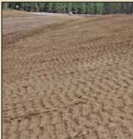
Figure 10.11 – Trackwalking creates imprints on the soil surface, but will also compact surface and subsurface soils.
