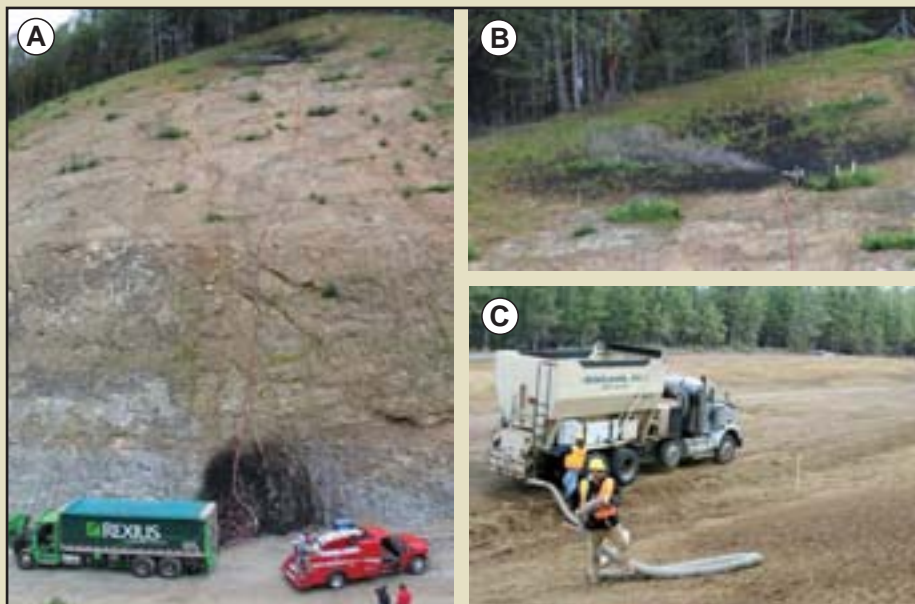
Figure 10.20 – Wood fiber mulch is applied on steeper slopes with mulch blowing equipment. Large trucks can hold between 75 and 100 yards of mulch (A) while smaller trucks can hold up to 25 yards (C). Mulch is pneumatically delivered to the site through an application hose which can reach several hundred feet up steep slopes (A) with still enough force for ample delivery of mulch (B).
