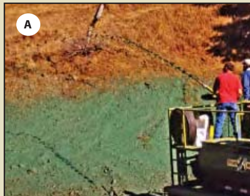
Figure 10.106 – High viscosity tackifiers, mixed at manufacturer recommended rates, keep the slurry together during application using a “stream” nozzle (A). Low viscosity tackifiers, or slurries with low concentrations of tackifiers, do not hold together when applied and will drift with wind (B) or run off slopes (C).
