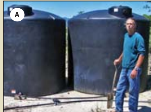
Figure 10.138 – Large holding tanks are used for temporary drip irrigation systems (A). A simple on/off valve controls water to the gravity-feed system (B). Pressure release valves (C) are used to control water pressure on hilly sites.
