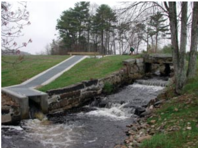
The completed fishway at the New Bedford Reservoir restores herring access to 200 acres of spawning habitat.
