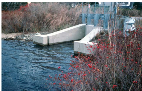
Pre-restoration: 48-inch culvert drains Little River, North Hampton, NH.
