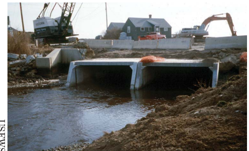
Post-restoration: twin 6-foot by 12-foot box culverts installed at Little River outlet.
