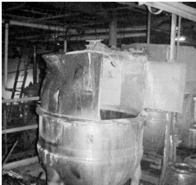
Figure A-2. Silver nitrate reactor on mezzanine 1 with open tank door (following explosion and fire).
