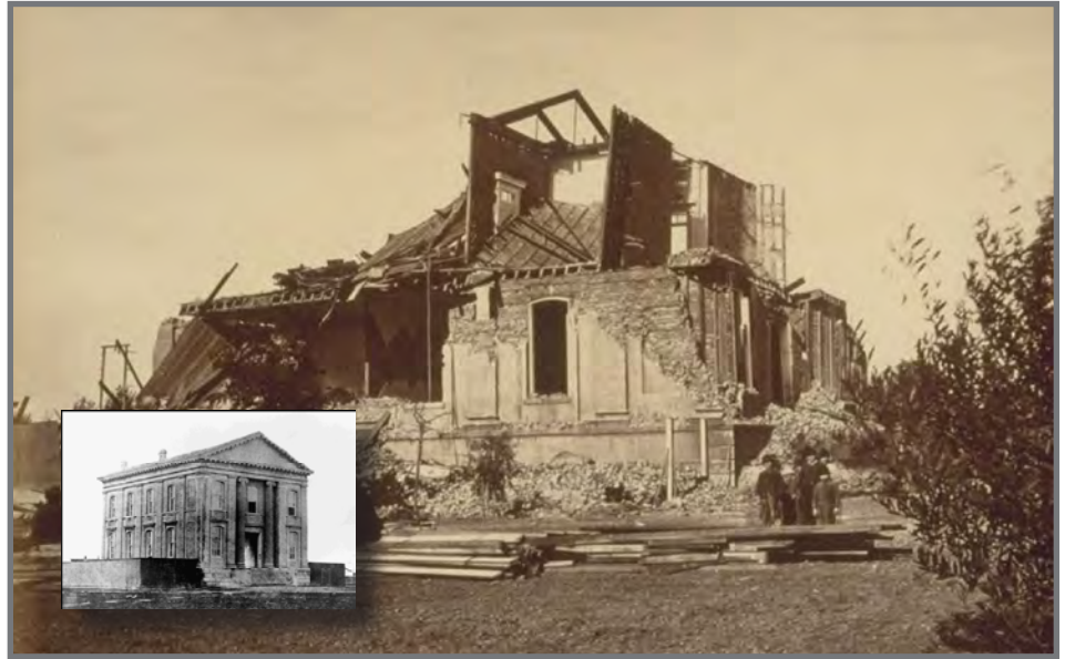
Strong shaking during the 1868 Hayward Fault earthquake caused the second story of the Alameda County Courthouse in San Leandro to collapse and severely damaged the building (photo courtesy of the Bancroft Library, University of California). The inset photo shows the building before the quake (photo courtesy of San Leandro Public Library). The 1868 quake devastated several East Bay towns and caused widespread damage in the San Francisco Bay region.
