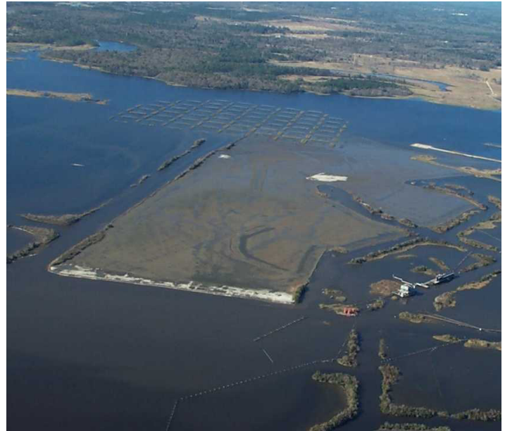
Completed Beneficial Dredged Material Project in Texas
