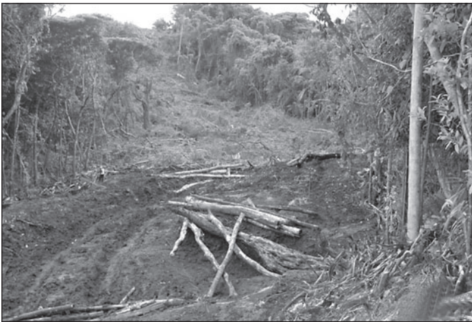
Figure 8: Compact Road at Beginning and End of Construction
