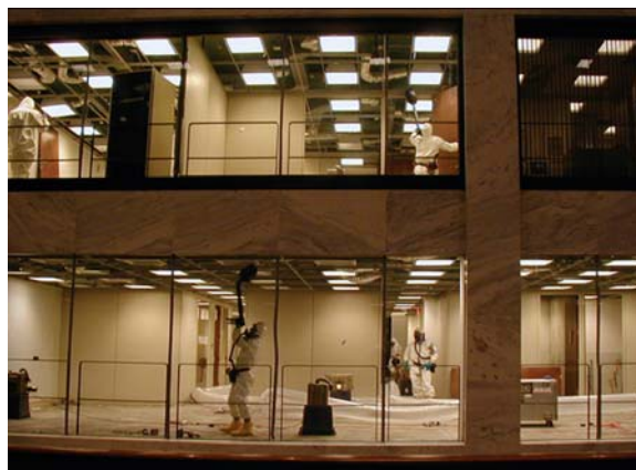
Decontamination crews in the Hart Senate Office Building in 2001.
