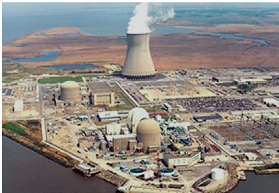
Hope Creek Nuclear Generating Station
