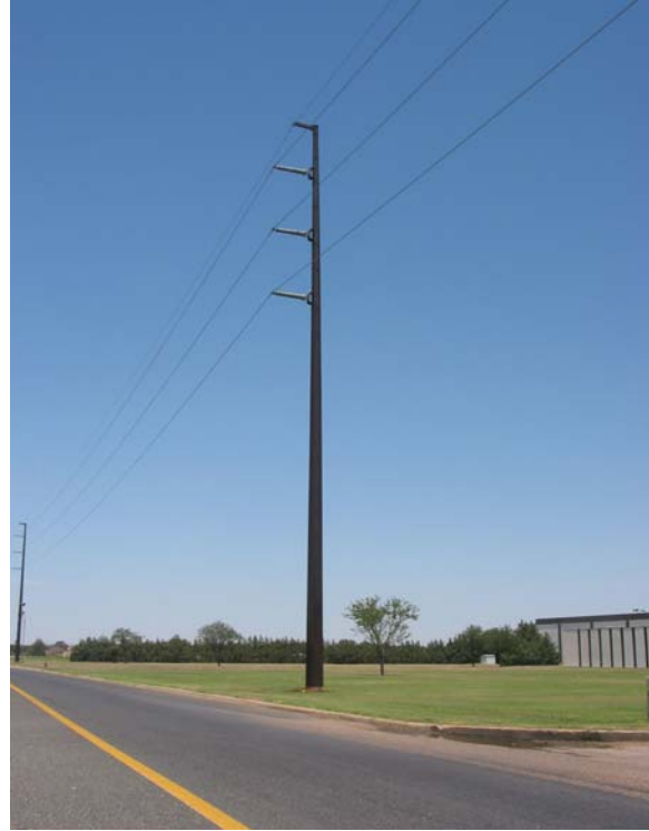
ETL: Single Steel Pole
