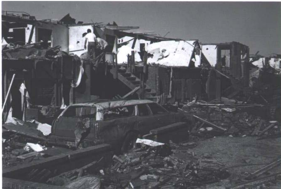
ACT: DOD 5: Most top story walls collapsed
