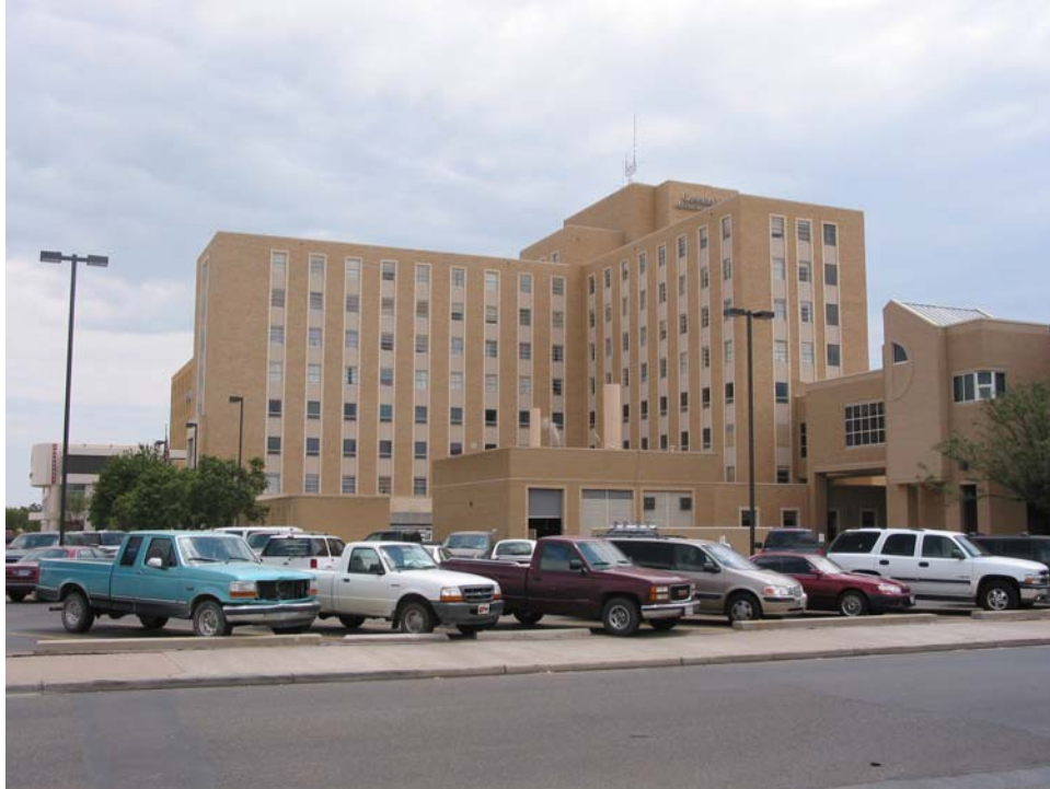
IB: Height from 1 to 10 stories; single-ply membrane, polyurethane foam, or metal roof systems; masonry, cut-stone or pre-cast wall panels; balconies, porches, or porticos; heavy façade; relatively small windows
