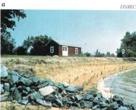
A fringe of marsh grasses as narrow as eight feet can reduce wave energy by over 50 percent (a—during planting; b—one year later).
