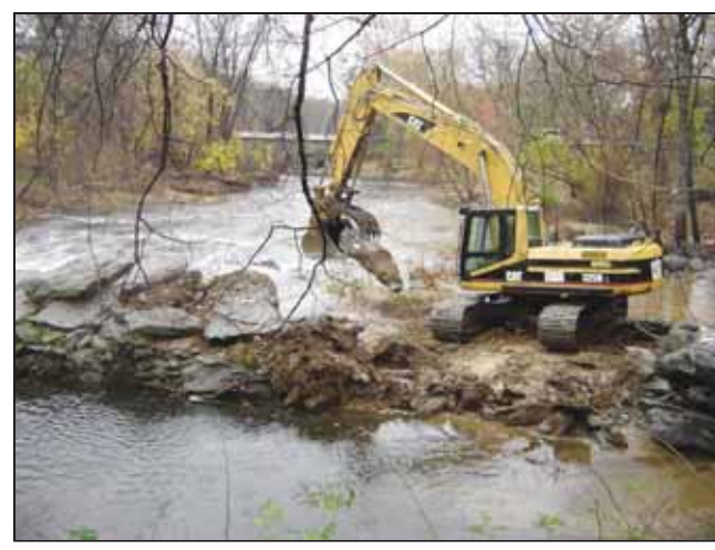
(Above) Breaking down the walls!
