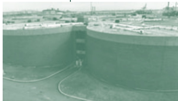
Northeast Water Pollution Control Plant
