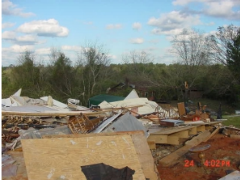
Mobile home blown off its foundation 10 miles northeast of Raleigh.
