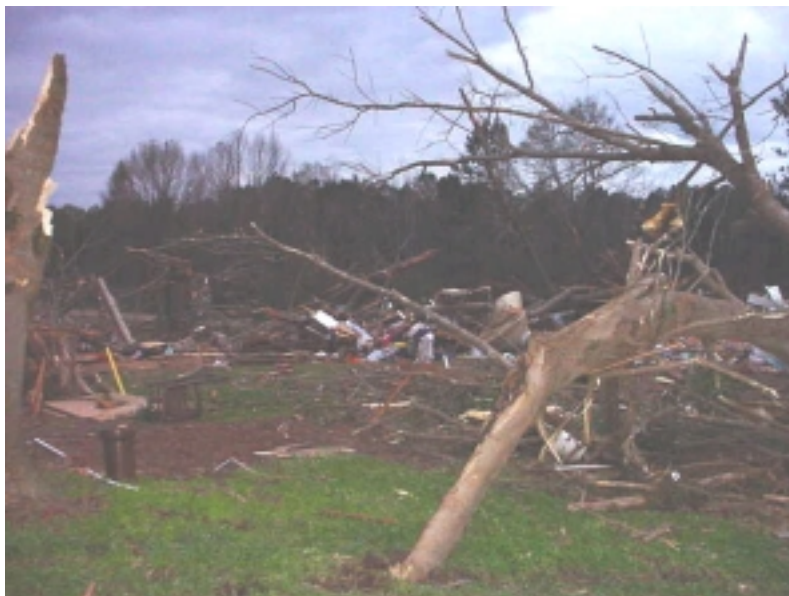
Destroyed home where one fatality and two injuries occurred.
