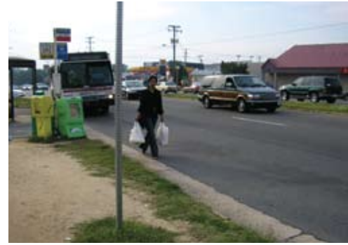
This shelter is not connected to a sidewalk system, so pedestrians must either travel in the road or grass to get to the bus stop. This is especially problematic for wheelchair users.
