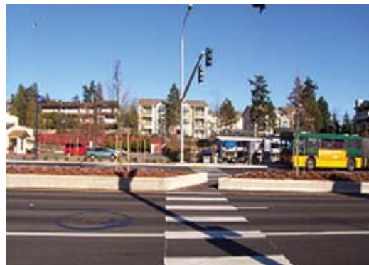
The median island near this transit stop includes an angled cut-through for pedestrians. This feature encourages pedestrians to face to the right and look for oncoming traffic before crossing.
