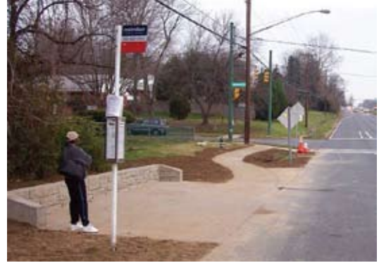
A level landing pad has been provided at this bus stop.
