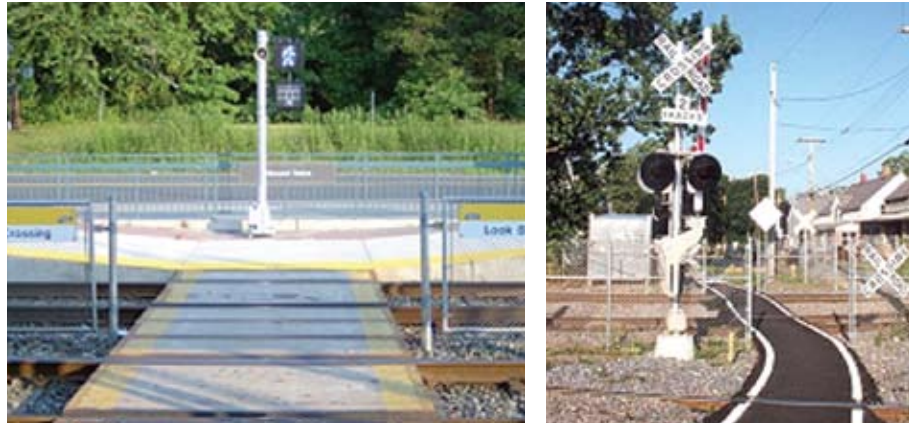
These pedestrian crossings illustrate many of the safety treatments that can be used at at-grade railroad crossings including: gates, warning stripes on the walkway, pedestrian walk signal similar to those used on roadways (left photo), flashing lights, warning signs and fencing (right photo). The pedestrian walkways are clearly marked and provide stable surfaces.
