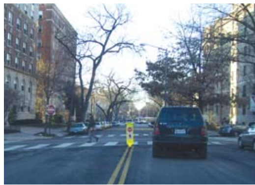
High-visibility crosswalks can be supplemented by “in-roadway pedestrian crossing signs” that remind drivers of state laws requiring them to yield or stop for pedestrians in the crosswalk. Pictured is a ladder type crosswalk marking, with an in-roadway pedestrian crossing sign.
