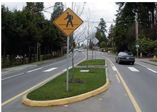
This roadway was modified from a four-lane, undivided roadway to two through lanes with a center turn lane and bicycle lanes. This change provided space to construct median islands and increase the safety of midblock crossings.
