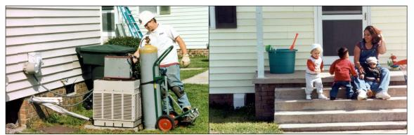
Thousands of family housing units on U.S. military bases like those at Marine Corps Base Camp Lejuene (pictured above) have been retrofitted with GHPs. At left, a construction worker discharges the refrigerant from an old heat pump in preparation for removing it. After installation, a small white box at foundation level (seen in the lower left corner of the photo at right) is the only outdoor evidence of a new GHP.
