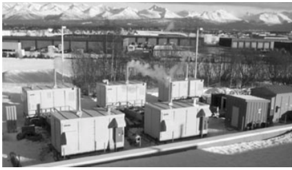
Figure 5. 200-kW phosphoric acid fuel cells.
