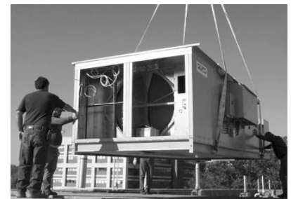
Figure 8. Desiccant/enthalpy dehumidifier.
