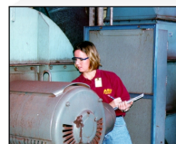
U.S. Postal Service Processing and Distributing Center, Atlanta, GA
