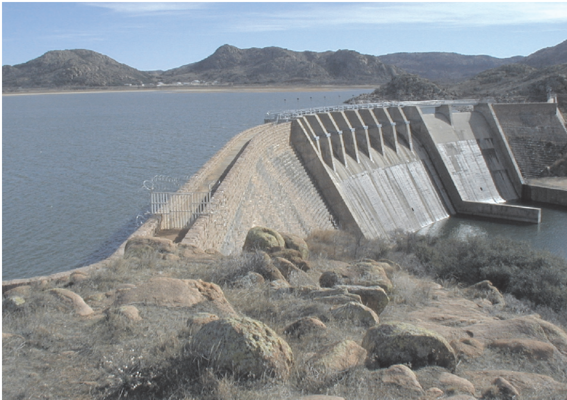
Photograph of Lake Altus dam taken by S. Jerrod Smith.
