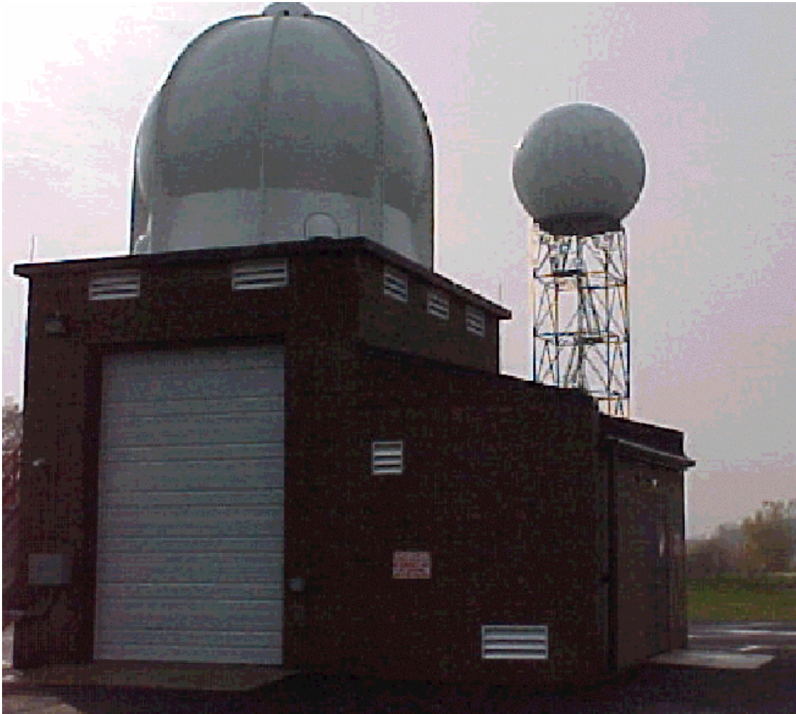
Figure B-2 - NWS Low-Bay Upper Air Shelter
