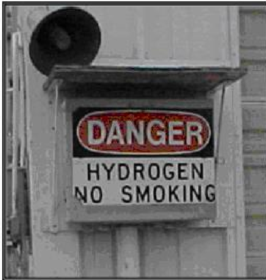
Figure B-10 - Closed Remote Control Panel with Rain Cover
