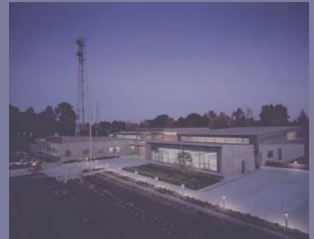
King County OEM Emergency Coordination Center
