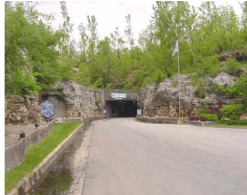
Entrance to cave housing NRC Space
