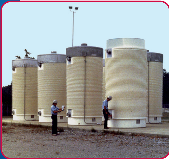
Dry Storage of Spent Nuclear Fuel
