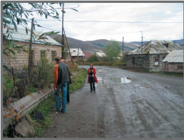
Photograph of the Armenia Road Project, which is in the process of procuring services to pave roads such as the local roads visited by OIG auditors.
