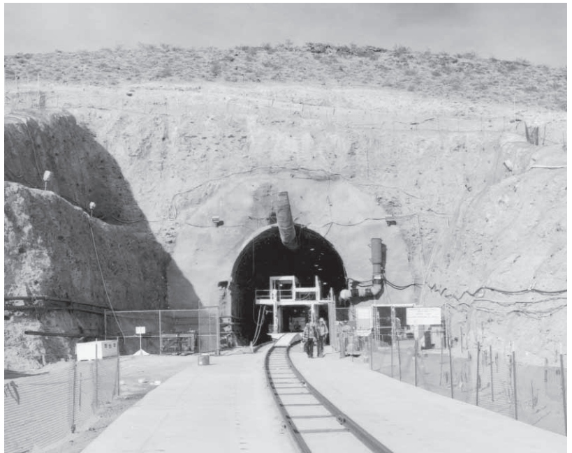
Starter tunnel at proposed Yucca Mountain site
