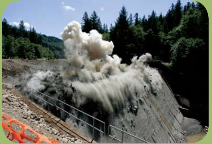
Demolition of the Marmot Dam on the Sandy River, Oregon, 2007.
