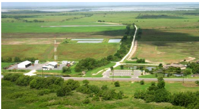
Aerial view of refuge facilities and moist soil units.
