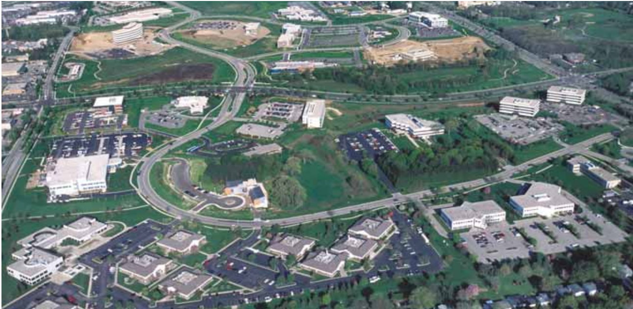
Research parks can be a boost for areas not known for technology. UW-M has helped build an entrepreneurial presence with its University Research Park, shown in this aerial view.
