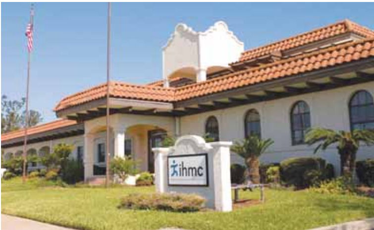
IHMC's headquarters in downtown Pensacola's historic district has helped to revitalize the surrounding area.
