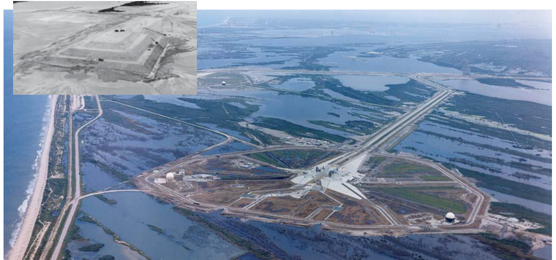
A sand pyramid, at top, was formed for the creation of a launch pad at KSC's Complex 39 on Merritt Island.
