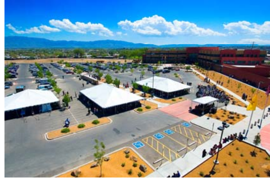
Aerial view of NIPTC
