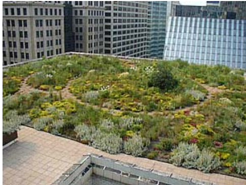
Chicago City Hall Urban Heat Island Initiative project (Source: Roofscapes, Inc. )
