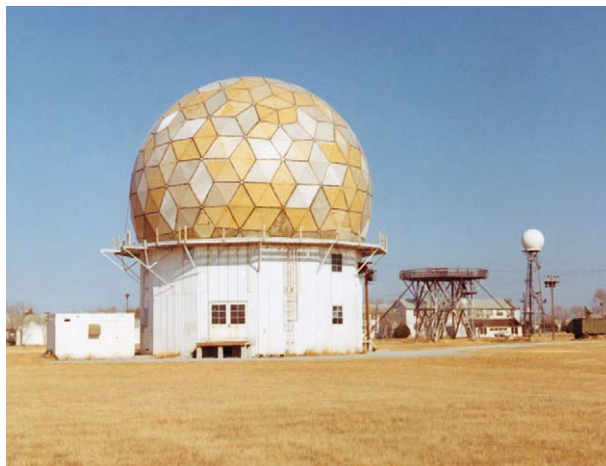
FIG. 6. The new (surplus) Norman Doppler radar building, with the open tower, research WSR-57 radar, and NSSL building in background. The building was later painted “NOAA blue” with the radome painted white. [NSSL photo.]
