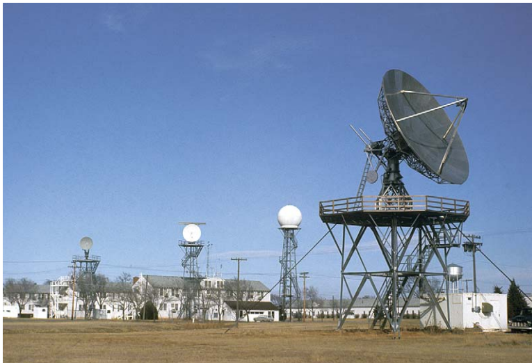
FIG. 5. (right) Norman 10-cm pulsed Doppler radar antenna and pedestal on an open tower with the transmitter in the building at the base (1969). (The decommissioned antenna and pedestal are now on permanent display at ground level on the same site.) The open tower was chosen as a cost-savings measure, but it proved to be unsatisfactory. So, the antenna and pedestal were subsequently moved to the permanent building shown in Fig. 6. The radar to the left of the tower was NSSL's/NSRP's WSR-57 research surveillance radar. The other two radars in the left part of the picture were used for aircraft tracking as part of Project Rough Rider. The two-story former Navy barracks building behind the three radars housed NSRP's Weather Radar Laboratory and then NSSL from 1962 through 1972. [NSSL photo.]
