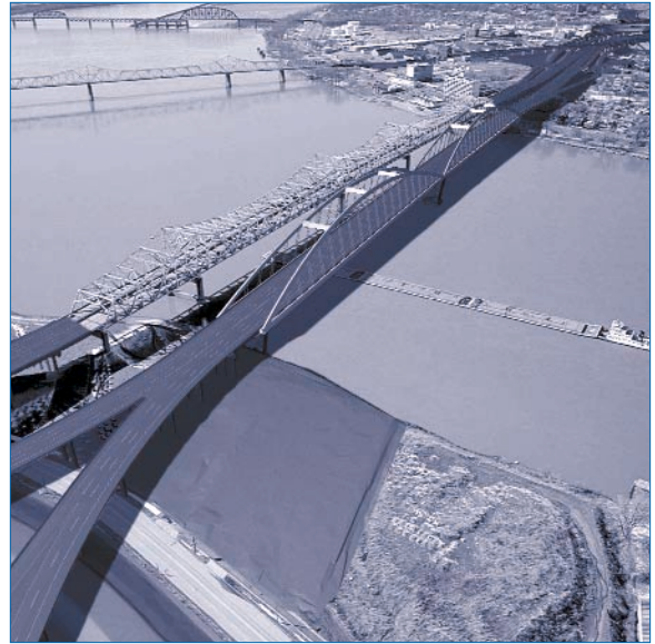
Louisville-Southern Indiana Ohio River Bridges Project Jefferson County, Kentucky and Clark County, Indiana
