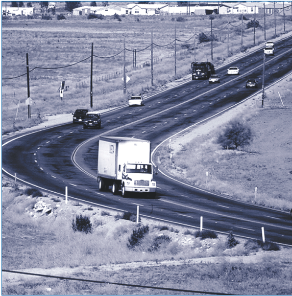
Community and Environmental Transportation Acceptability Process (CETAP), Riverside County, California
