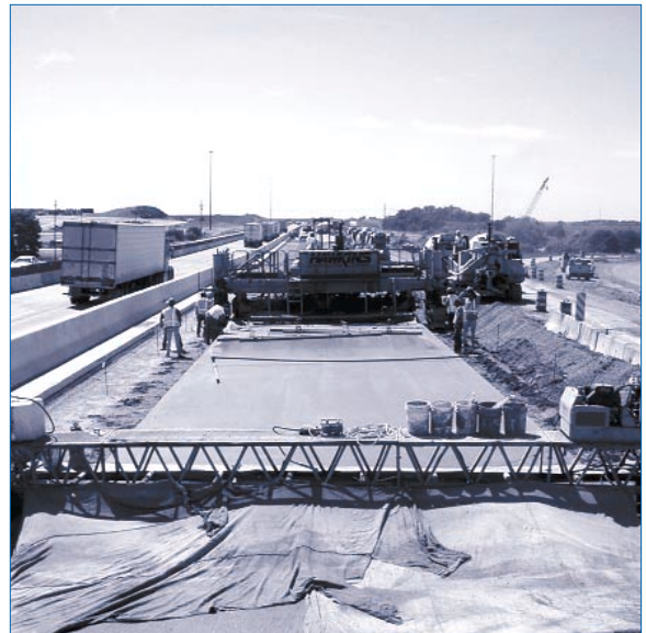
Interstate 80 (I-80) Upgrade, Lincoln-Omaha, Nebraska
